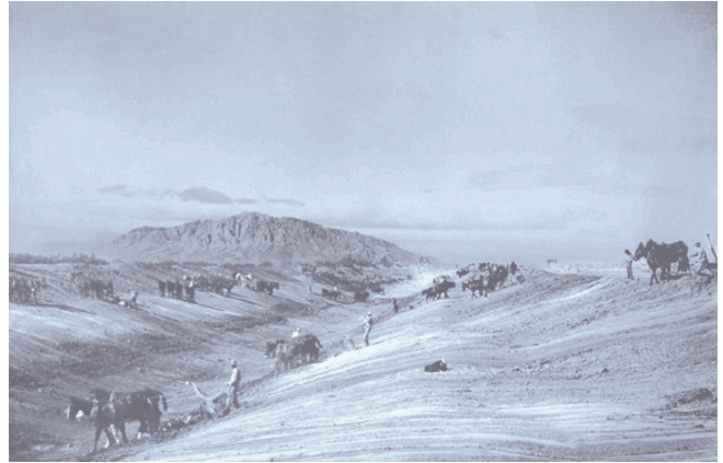
Early construction on the All American Canal
