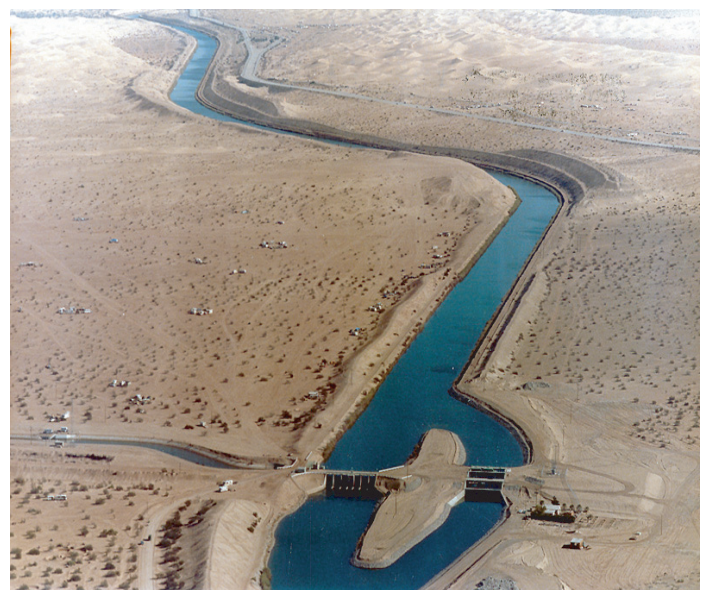
Aerial view of the All-American Canal
